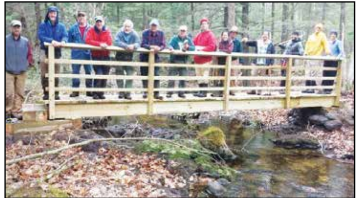
Volunteers stand on the newly completed bridge on the Metacomet-Monadnock trail in Troy, N.H.
