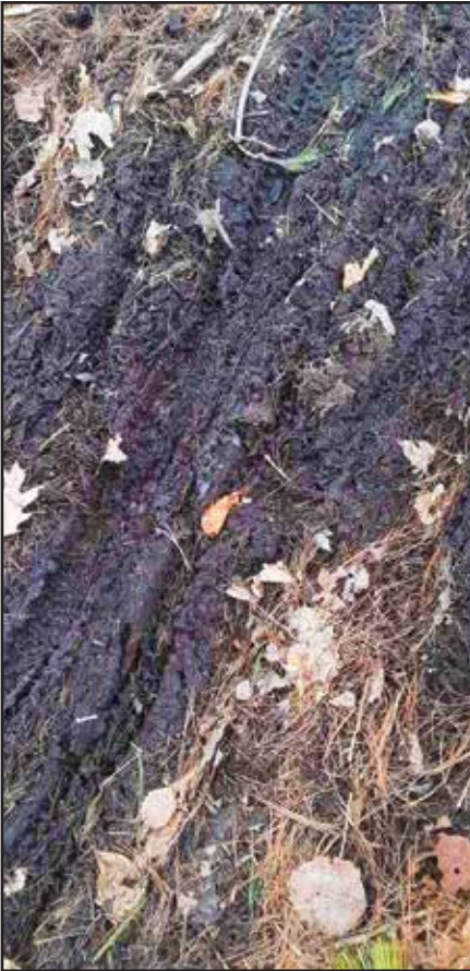
Photo by: Richie Holstein. Bikes create long trenches through muddy spots on a trail and can create damage that is hard to repair.
