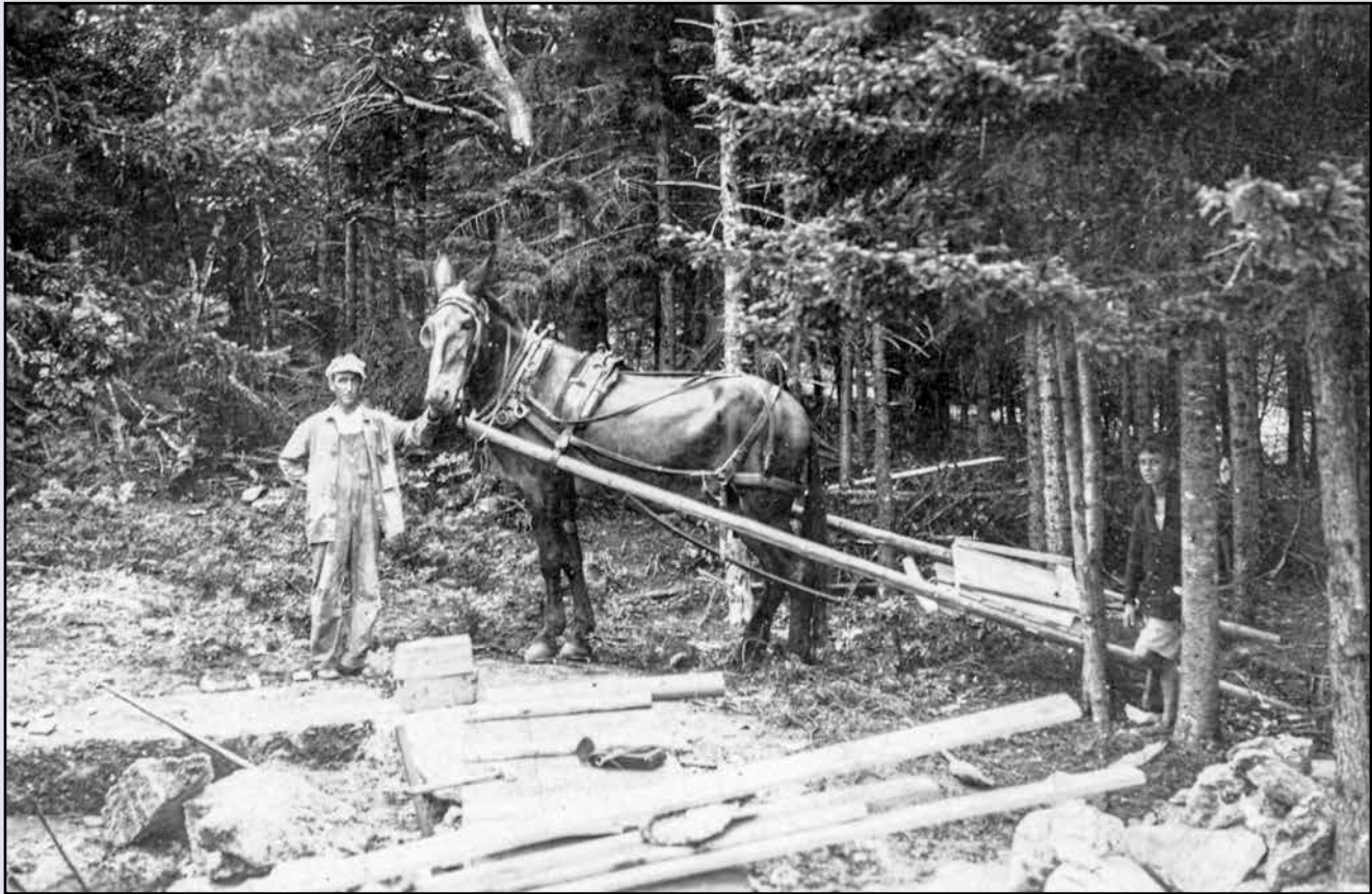
Mary, the mule, hauling supplies to build Hi Cabin. A tractor was also used, but it kept breaking down. AMC Archives.
