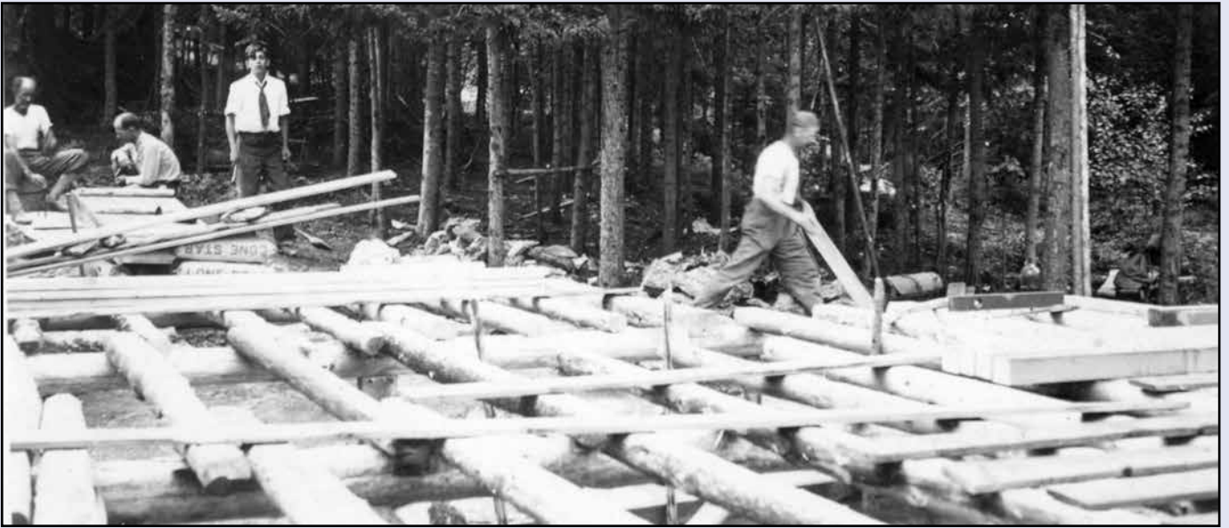
August 7, 1931: Construction has started laying the foundation and the beams for the floor. AMC Archives.
