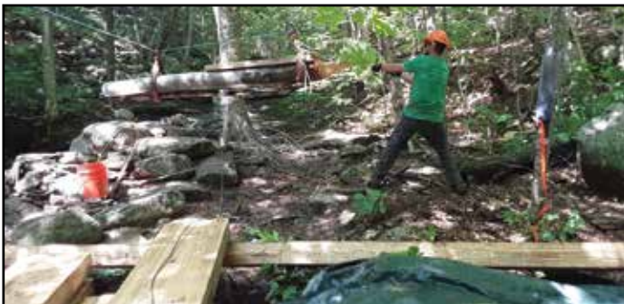
Keith guides the old stringer out of the way.
