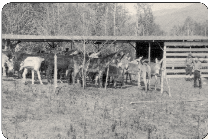
Burros used to haul construction materials were stabled near Appalachia Trailhead.
