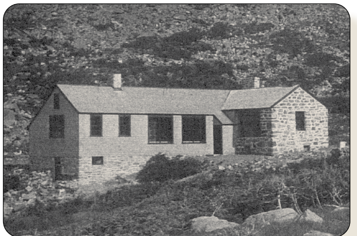
Hut #3 was originally constructed in 1922 as a dormitory to accommodate 36 men and 24 women. In 1929 the hut was expanded to add a kitchen and dining area and a bedroom for the Hut Master. These photos show the stages of the construction and the finished hut.
