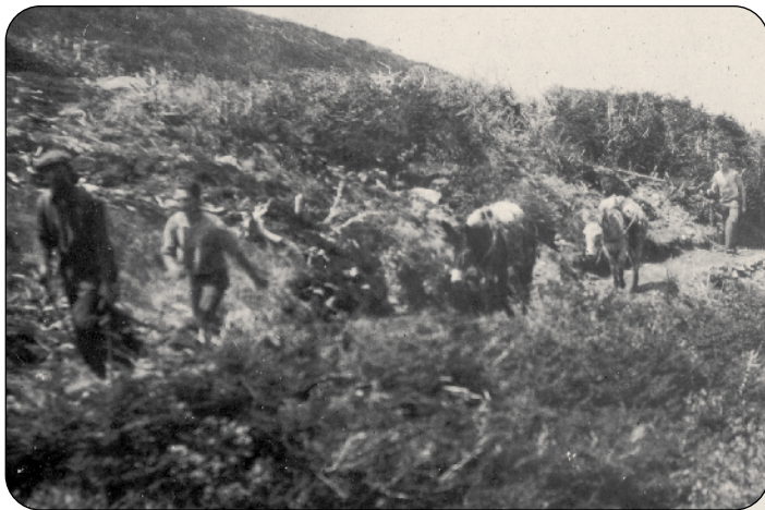
A string of burros could haul over half a ton from the valley to the construction site at Madison Spring Hut in under four hours and do it over and over.
